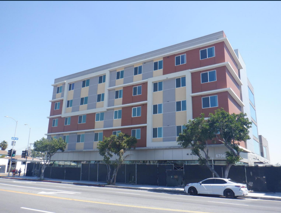
View from across the street at 6706 S Main St.
